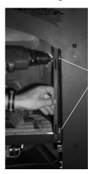
Door Bracket attaches with 2 screws.
